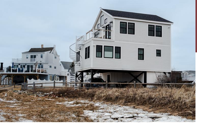
This home on Plum Island is crafted to meet environmental standards, including the Massachusetts Wetlands Protection Act. Elevated on piers two feet above FEMA flood levels, it is designed to withstand storms and support dune dynamics and native vegetation growth. The surrounding pea stone and sand surfaces enhance groundwater health and stormwater management.
