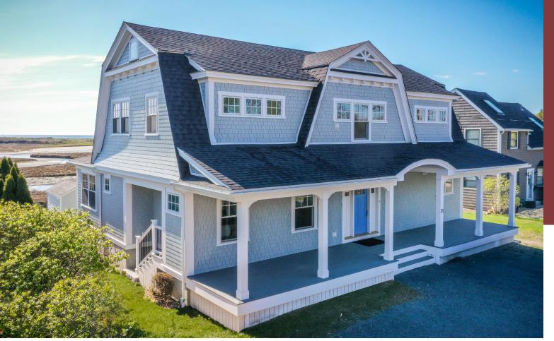
This new construction project, overlooking Good Harbor Beach is a classic Shingle Style home featuring a gabled roof with a substantial roof rake. The exterior facade is enhanced by a trim break with ornamental corbels and a flared skirt, adding elegant detail.
