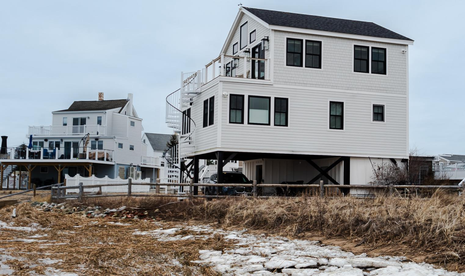
*This home on Plum Island is crafted to meet environmental standards, including the Massachusetts Wetlands Protection Act. Elevated on piers two feet above FEMA flood levels, it is designed to withstand storms and support dune dynamics and native vegetation growth. The surrounding pea stone and sand surfaces enhance groundwater health and stormwater management.*
